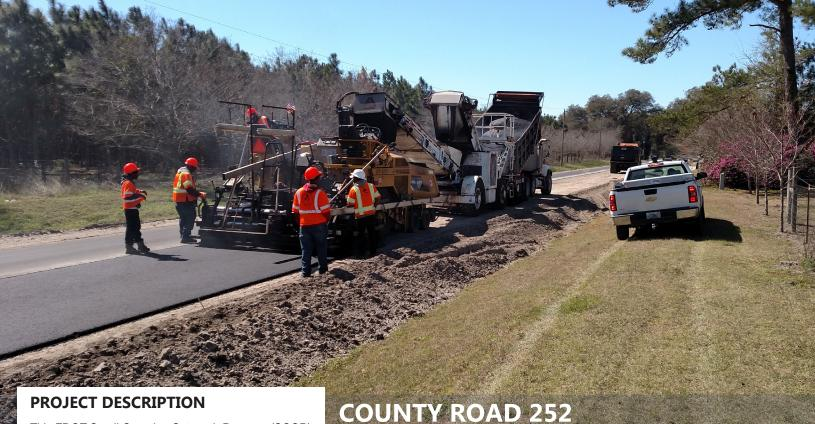
This FDOT Small Counties Outreach Program (SCOP) funded project consisted of reclaiming, widening, and resurfacing 10.01 miles of existing pavement from SR 51 east on CR 252 to SR 249/US 129. This project also consisted of constructing cross drains with end treatments, grassing all disturbed areas, and replacement of all signs within project limits.
