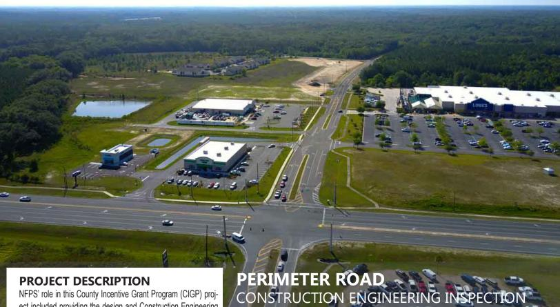
NFPS' role in this County Incentive Grant Program (CIGP) project included providing the design and Construction Engineering Inspection (CEI) of the stabilizing and paving of an existing dirt road, and adding a new roadway between US Hwy 90 and NE 72nd Trace. This also consisted of 24-foot paved roadway surface, grassed shoulders, and roadside ditches. The total length was 2.5 miles of Perimeter Road, a new alignment through the woods in Live Oak, Florida.
