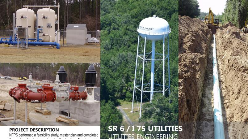
NFPS performed a feasibility study, master plan and completed the engineering design and cost estimates for a County-owned and operated potable water supply and distribution system and a 125,000 gallon per day (GPD) modular waste water treatment plant that can be expanded in quarter increments up to a 500,000 GPD capacity. The project also included a 19.17-acre effluent spray field to serve the Phase 1 Planning Area along SR-6 East and West of the I-75/SR-6 intersection (Exit 460).
